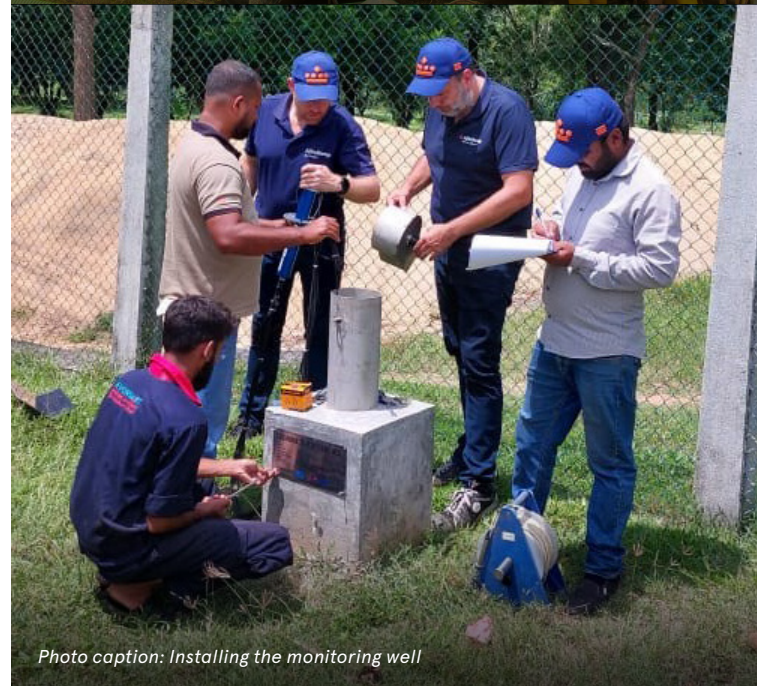
Photo caption: Drilling for the monitoring wells
